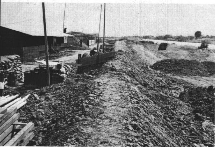
BERM BUILDING —Earthen berm shown under construction is typical of fortifications at Special Forces camps.
