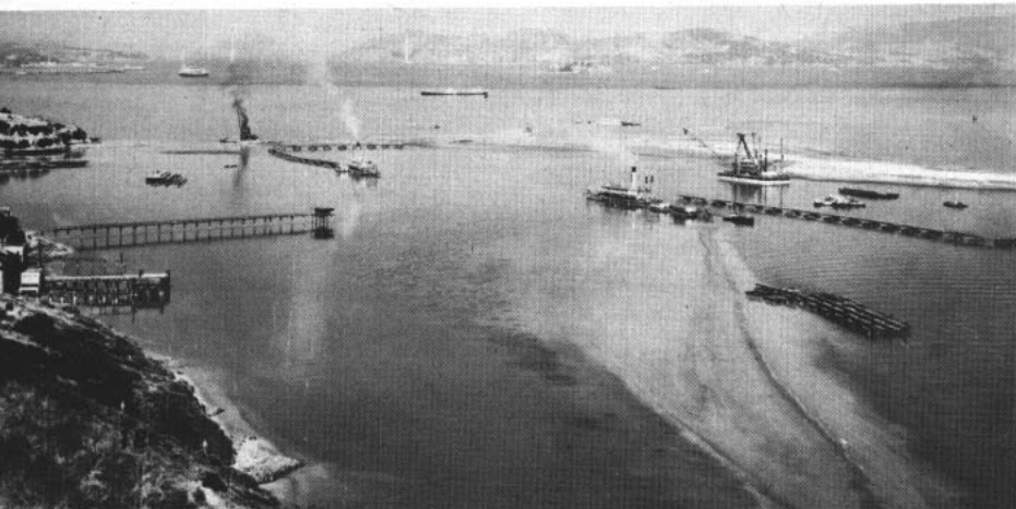
BUILD UP —Dredges dig up bottom of San Francisco Bay to build an island.
