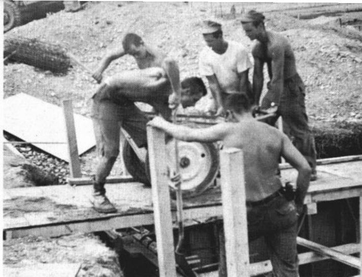
LINE WORK —Seabees pour concrete for reinforced bunker at U. S. Special Forces camp up front in Vietnam.
