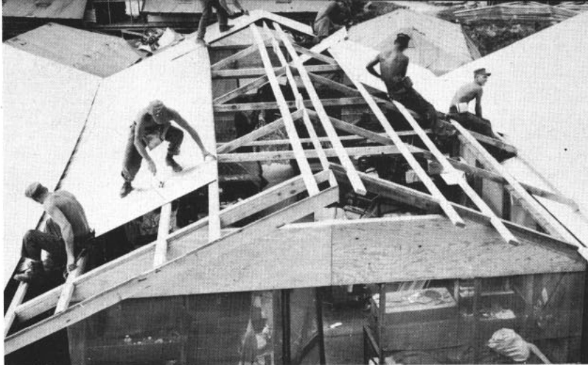
ON A TIN ROOF—MCB One works on quarters for Marines at Da Nang.
